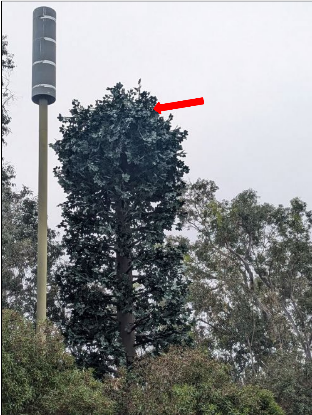
Figure 3: Monopine indicated by red arrow (Source: Applicant Photo; annotations for red arrow by TLF).
