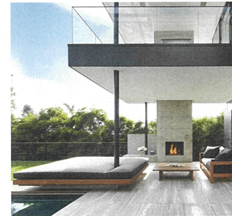
CLADDING - MIXTURE OF OFF-WHITE ACRYLIC STUCCO / FREE FORM NATURAL STONE / MATTE BLACK FASCIA METAL
