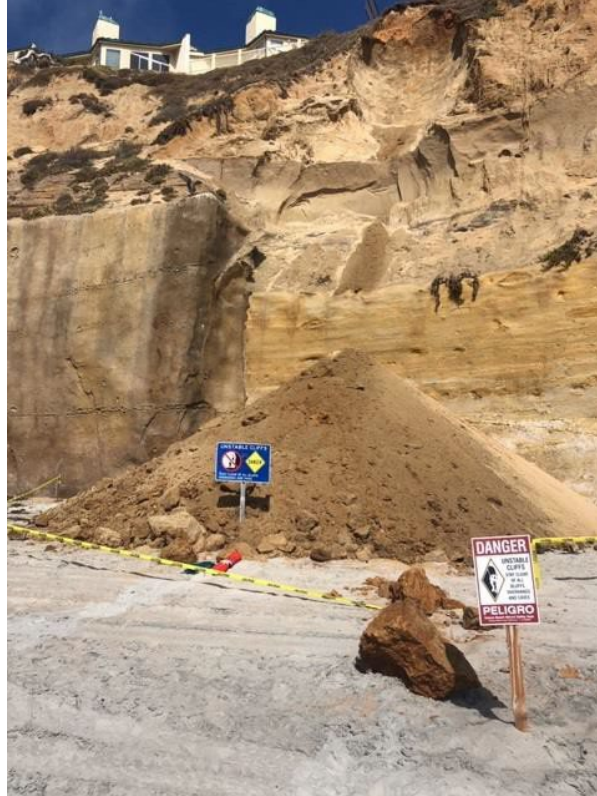
Figure 4-3 Bluff Collapse in Solana Beach September 13, 2019
