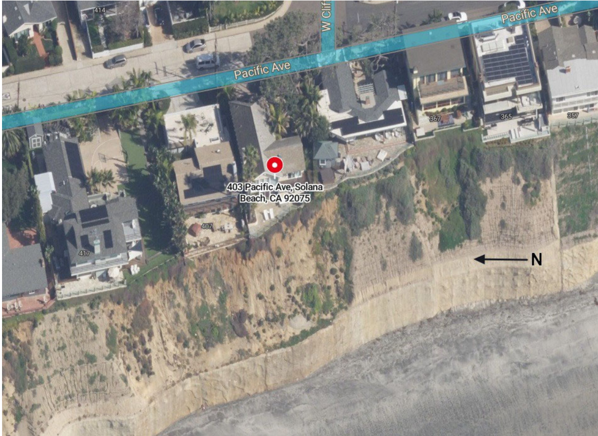
Figure 1. Subject site, seawall, and adjacent properties in 2022.
