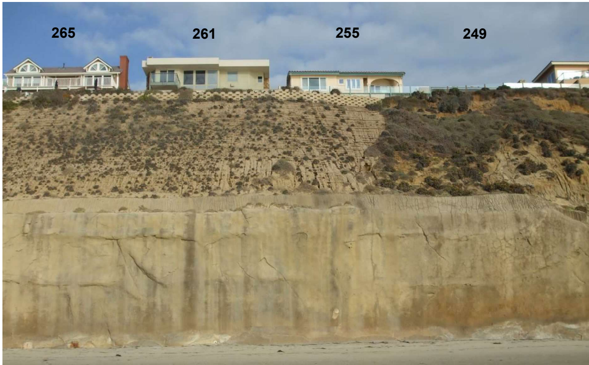
Photo 11: Upper bluff below 265 to 249 Pacific Avenue (November 4, 2013).
