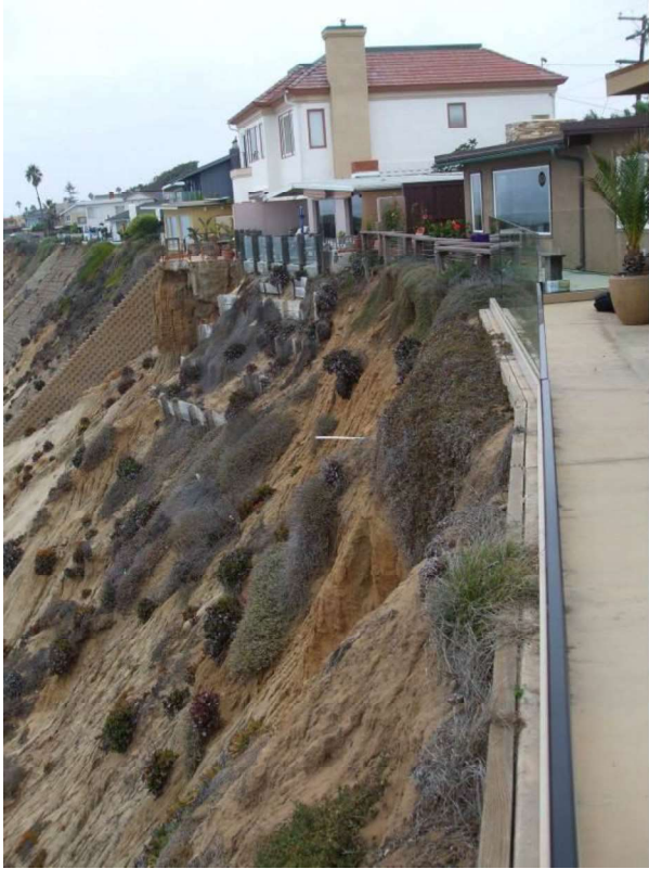
Photo 31: 311 Pacific Avenue looking north (November 4, 2013).
