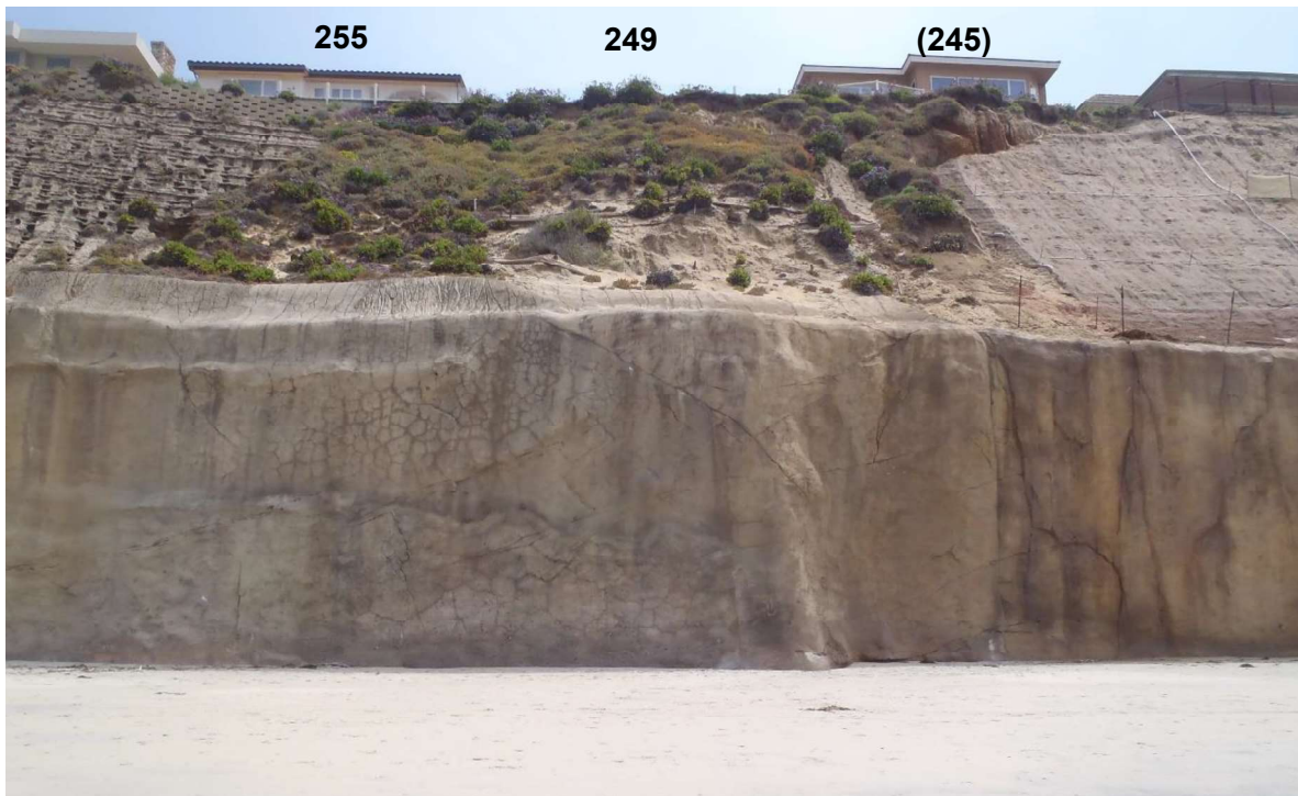
Photo 16: Upper bluff below 255 to 249 (& 245) Pacific Avenue (April 26, 2023).
