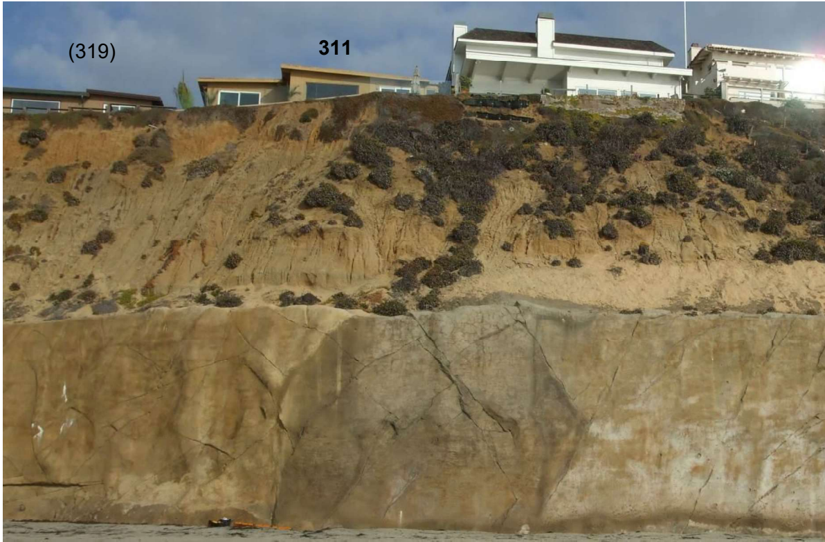
Photo 7: Upper bluff below 311 to 309 Pacific Avenue (November 4, 2013).
