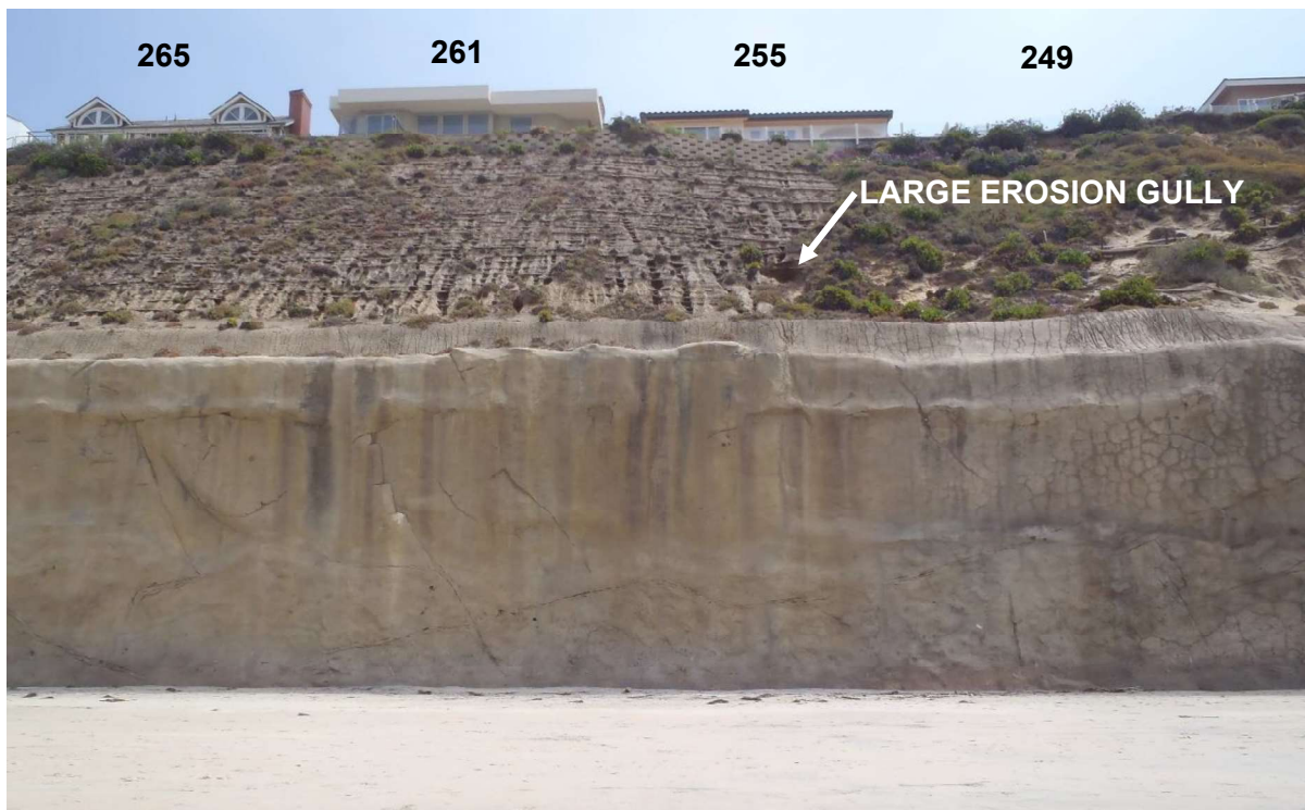
Photo 12: Upper bluff below 265 to 249 Pacific Avenue (April 26, 2023). Geogrid-reinforced slope is showing continued rill erosion due in part to lack of vegetative cover.
