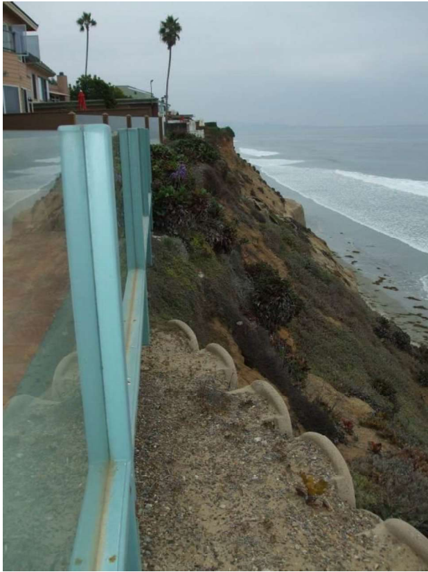
Photo 19: 255 Pacific Avenue looking south (November 4, 2013).
