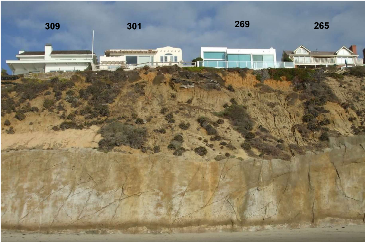
Photo 9: Upper bluff below 309 to 265 Pacific Avenue (November 4, 2013).
