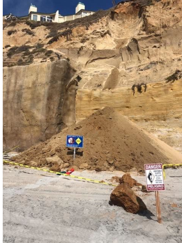
Figure 4-3 Bluff Collapse in Solana Beach September 13, 2019
